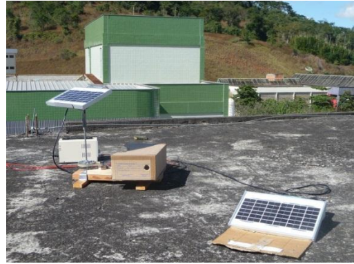
Figure 26 – Panels with same tilt.
